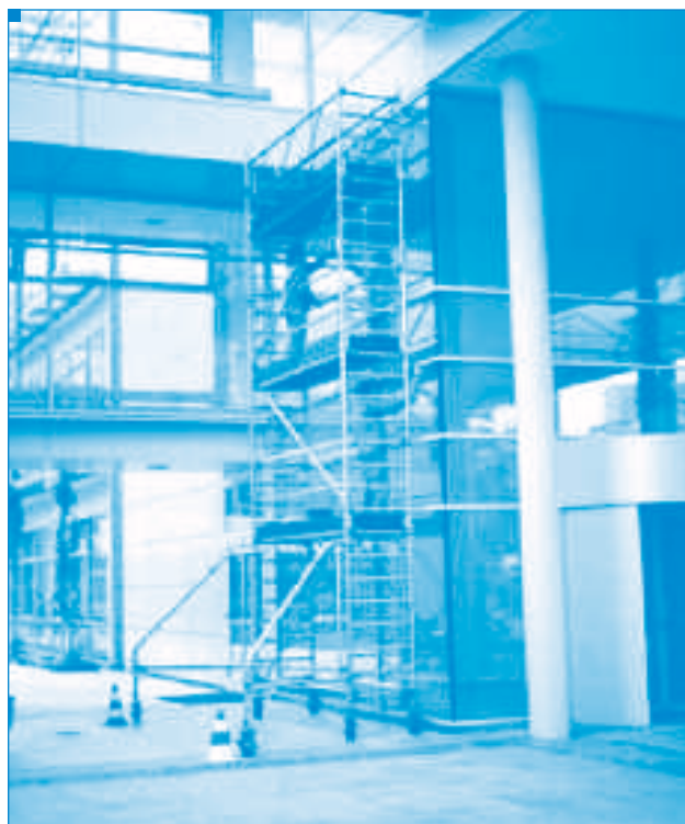
Example 3: Cleaning glass atria and roofs from the inside using a mobile elevated work platform (MEWP) – scissor or a vertical telescopic lift
