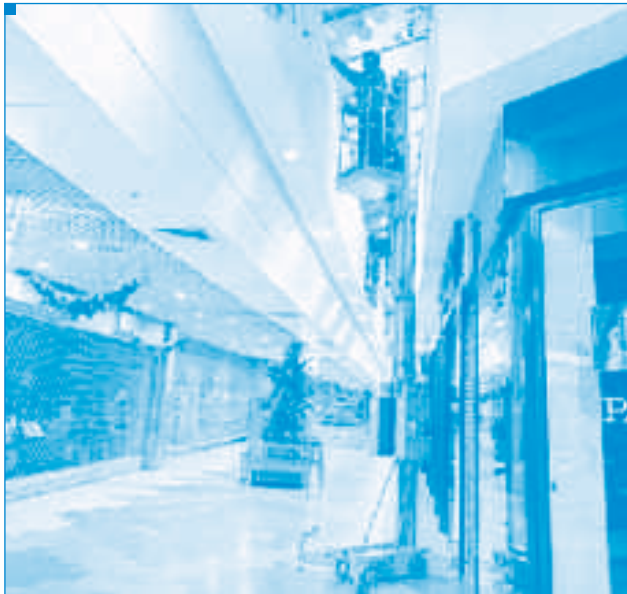
Example 4: Cleaning glass atria and roofs from the inside using a mobile elevated work platform (MEWP) with boom
