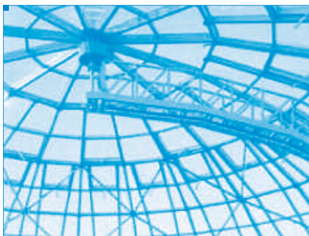
Example 2: Cleaning glass atria and roofs from the inside using a tower scaffold
